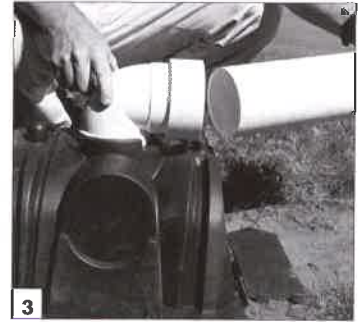
Connect inlet pipe.
