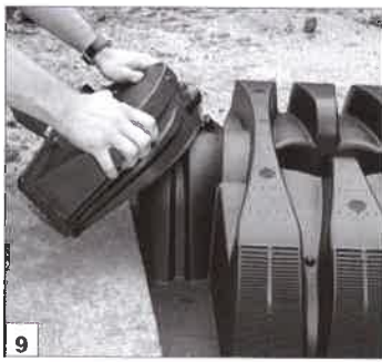
Place end cap outlet end.
