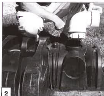
Insert Quick4 Plus Periscope.
