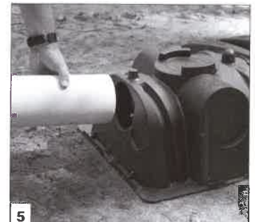
Insert inlet pipe.
