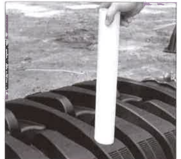
Chamber inspection port.
